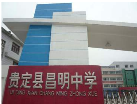
小組現正資助的貴定縣昌明中學。 Chang Ming Secondary School currently under CEA's subsidy.
