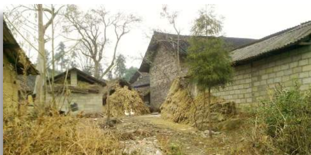
● 貴定縣農村的房屋。 Huts in villages in Guiding County.
