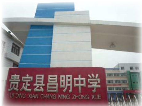
小組現正資助的貴定縣昌明中學。 Chang Ming Secondary School currently under CEA's subsidy.
