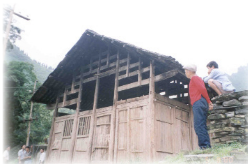
白岩村小殘破簡陋，小組遂援建以改善白岩村和排沙村學生的學習環境。 Reconstruction of Bai Yan Primary School helped improve the learning environment for students from two villages.
